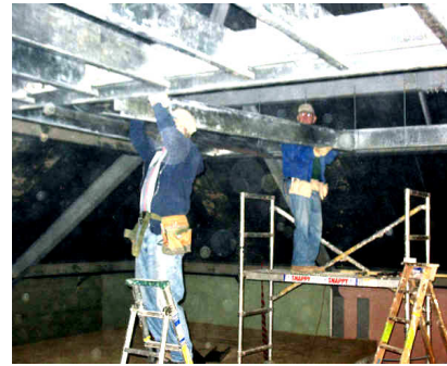
Don and Ed installing steel beams
